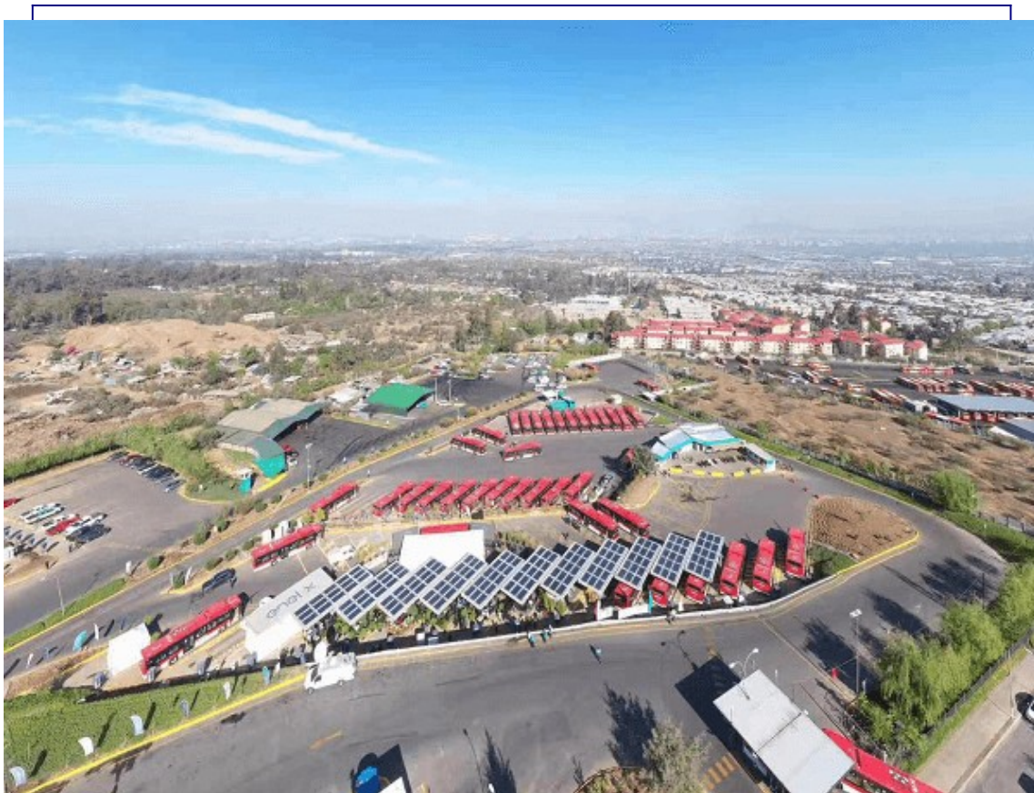
Figure 3: The new electric terminal at Peñalolén
