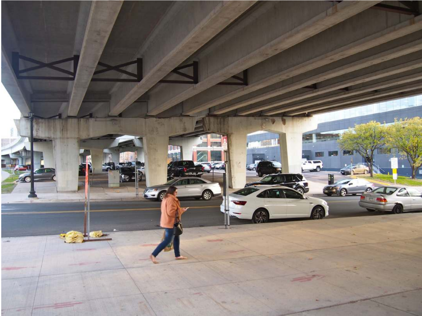
Figure 145: Existing raised I-94 viaduct in the North Loop
