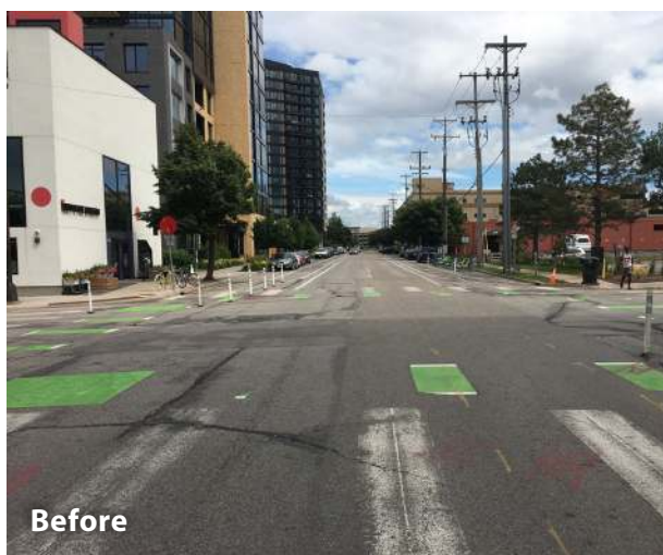
Figure 26: Paint and bollards improve conditions for people walking and bicycling; 11th Avenue and 2nd Street S
