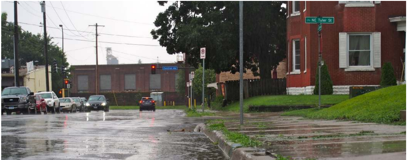
Figure 156: Incorporating stormwater infrastructure on street projects will help with localized flooding issues
