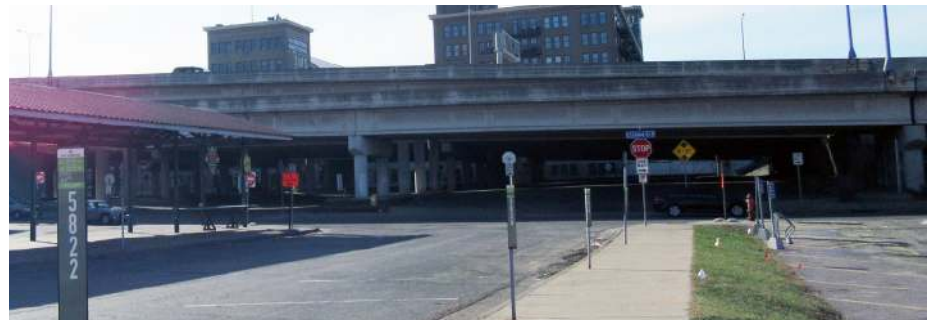
Figure 41: New 5th Street pedestrian bridge over I-35W
