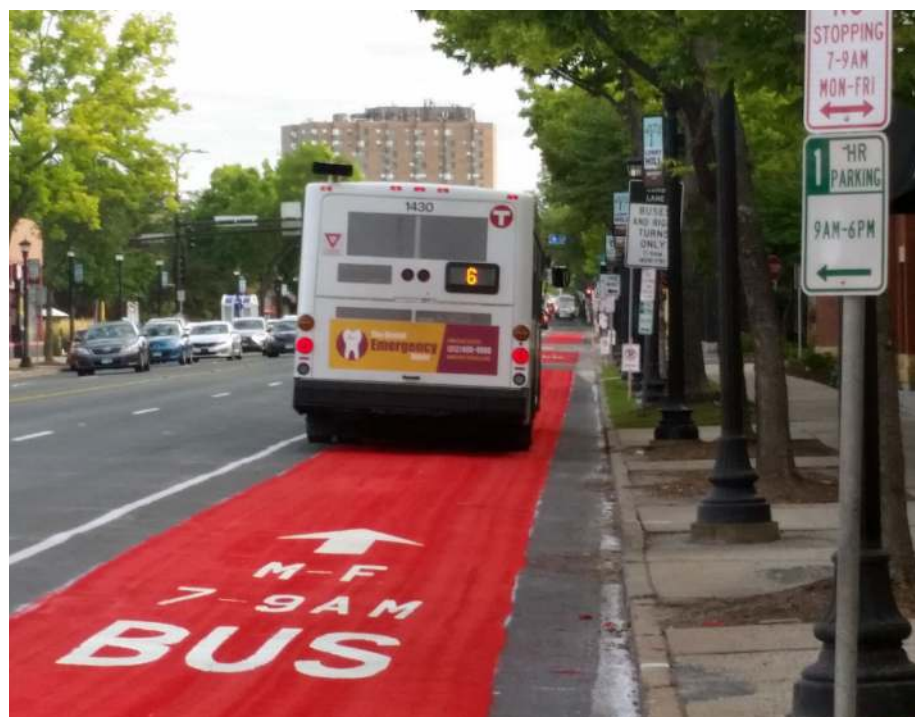
Figure 78: Painted bus lane
