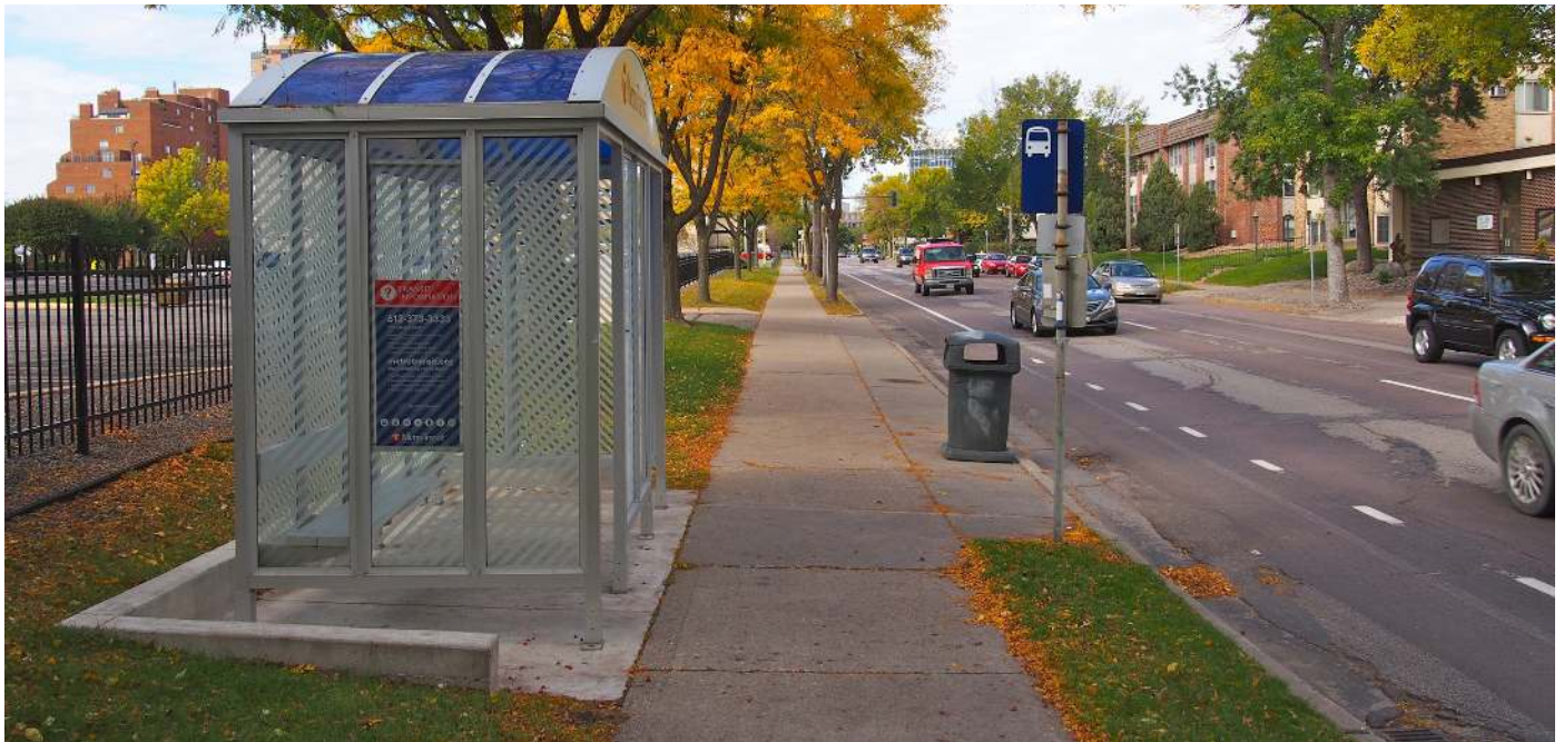
Figure 88: Well maintained transit stop
