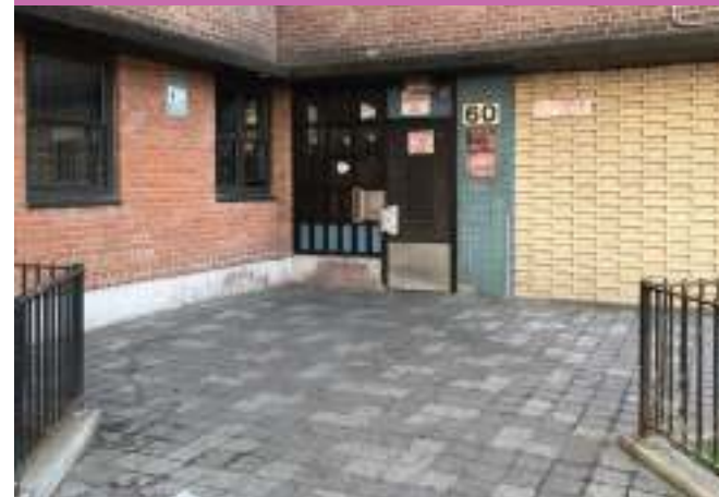
Paving at Baruch Houses, where subtle changes in the scoring of concrete provides visual differentiation and highlights building entrances.
