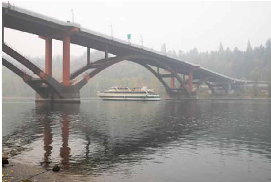
Figure 43 - Photo of the rebuilt Sellwood Bridge during the 2020 September wildfire smoke event. Photo – Motoya Nakamura, Multnomah County Communications.
