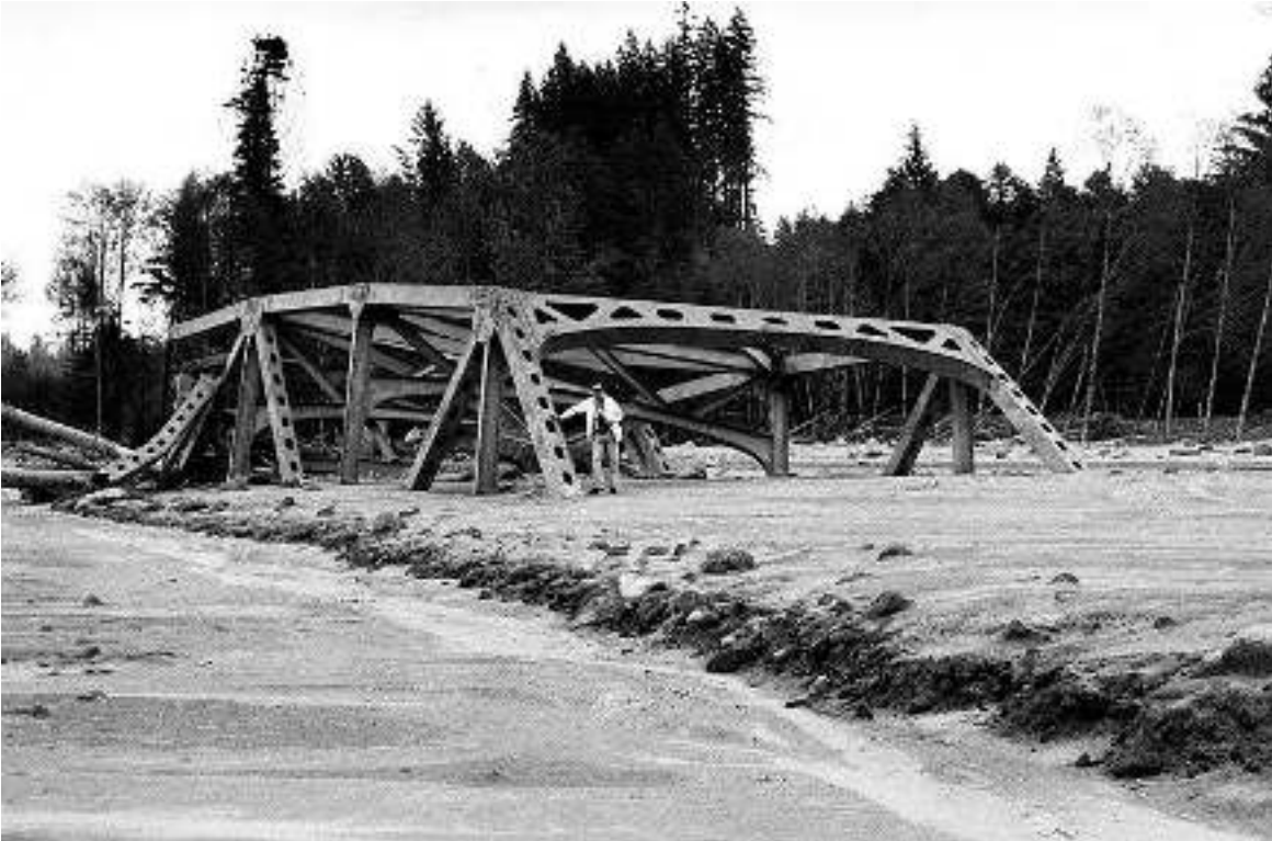
Figure 85 - The Saint Helens Bridge on Highway 504 in Washington was carried over a quarter mile downstream by a lahar from the 1980 Mount St. Helens eruption. Photo by R.L. Schuster for the United States Geological Survey.
