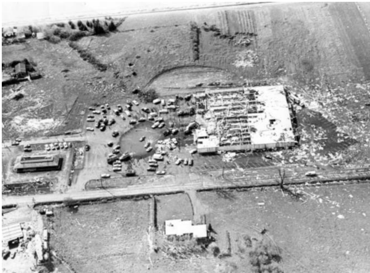
Figure 80 - Damage in Vancouver, Washington caused by the 1972 tornado. Photo and oral recount provided by Clark History.
