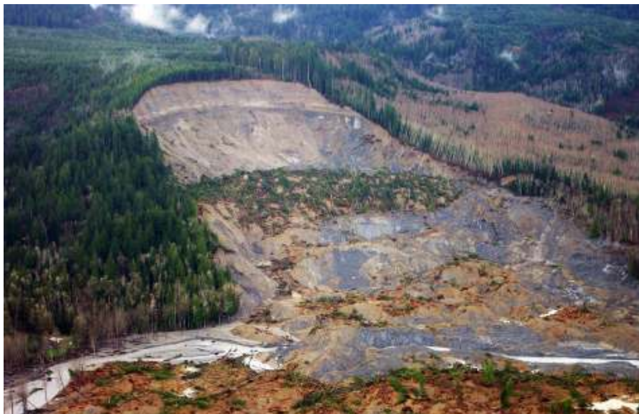
Figure 73 - 2014 Oso Landslide photo. Photo Jonathan Godt, US Geological Survey
