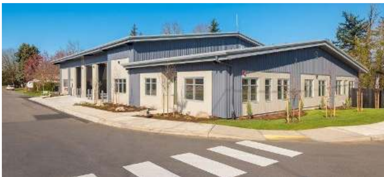
Figure 116 - New Fairview Public Works building. Photo from P&C Construction .
