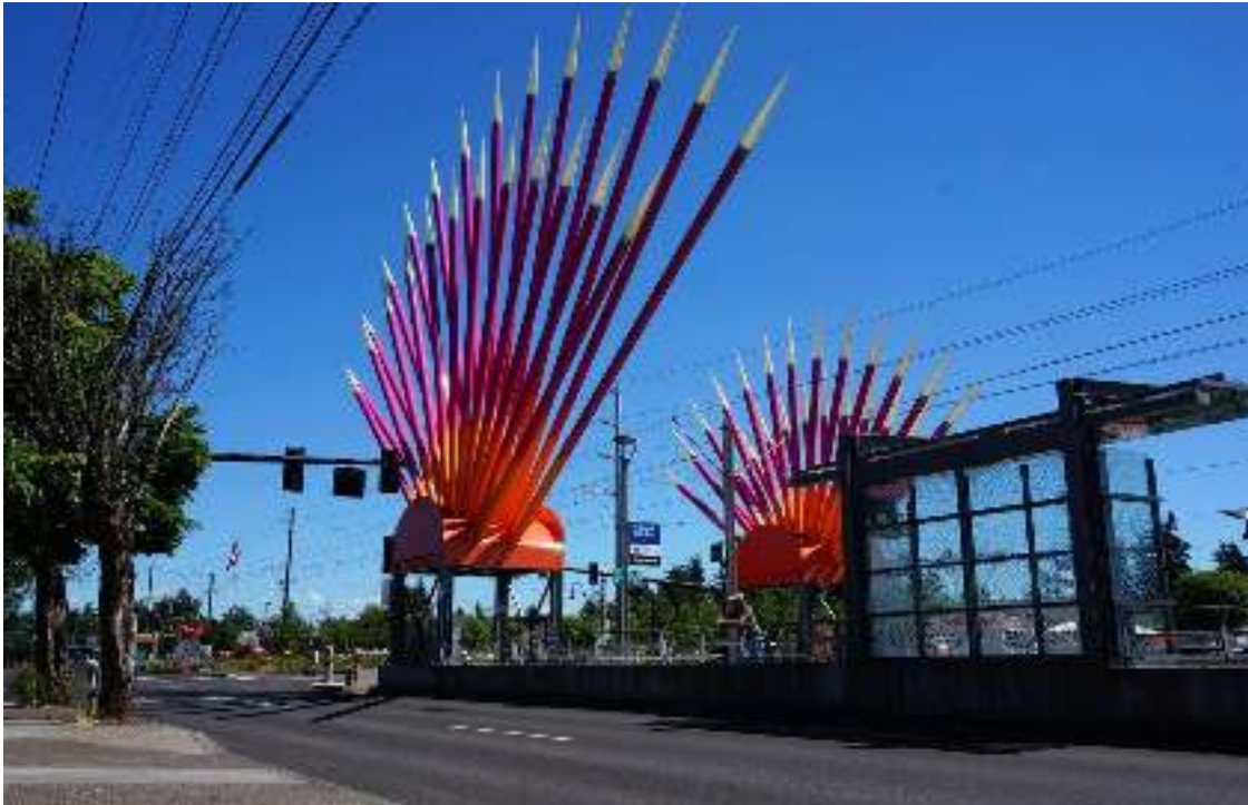
Figure 124- Public art at the Rockwood light rail station in Gresham. Photo - Metro
