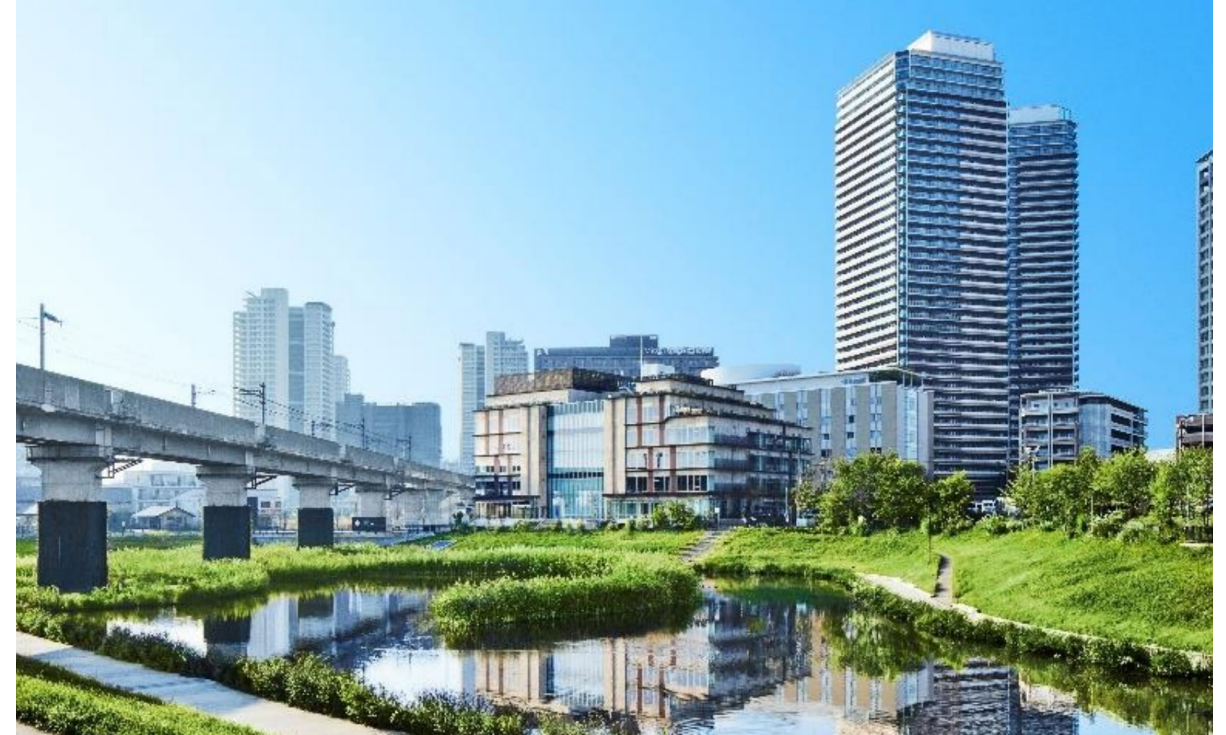
KOIL 2, Kashiwa no Ha, Chiba Prefecture LEED ND Platinum Certified Smart City
