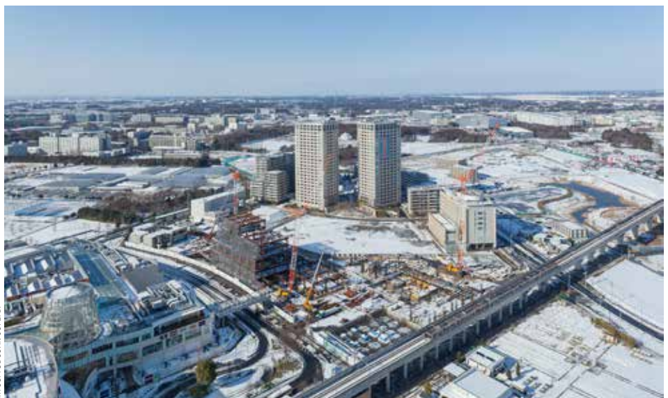
West side of Kashiwanoha Campus Station (parcels 147, 148, and 150) in January 2013.
