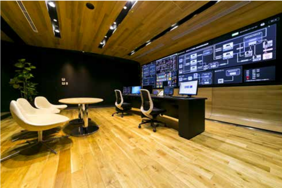
The Smart Center is on the second floor of the Mitsui Garden Hotel building.
