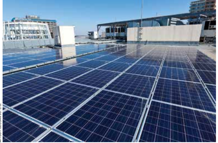
Energy from solar panels such as these installed on the roof of LaLaport Kashiwanoha—along with energy from storage cells, biogas cogeneration, and other sources, as well as TEPCO—is shared across parcels via private transmission lines, enabling a 26 percent reduction in electricity consumption during peak hours.
