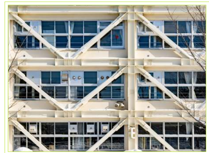
Steel seismic retrofit detail. Source: eSUB
