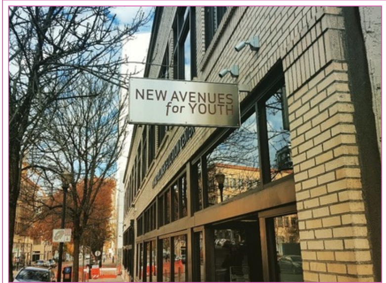
New Avenues for Youth building. Source: ECA PDX
