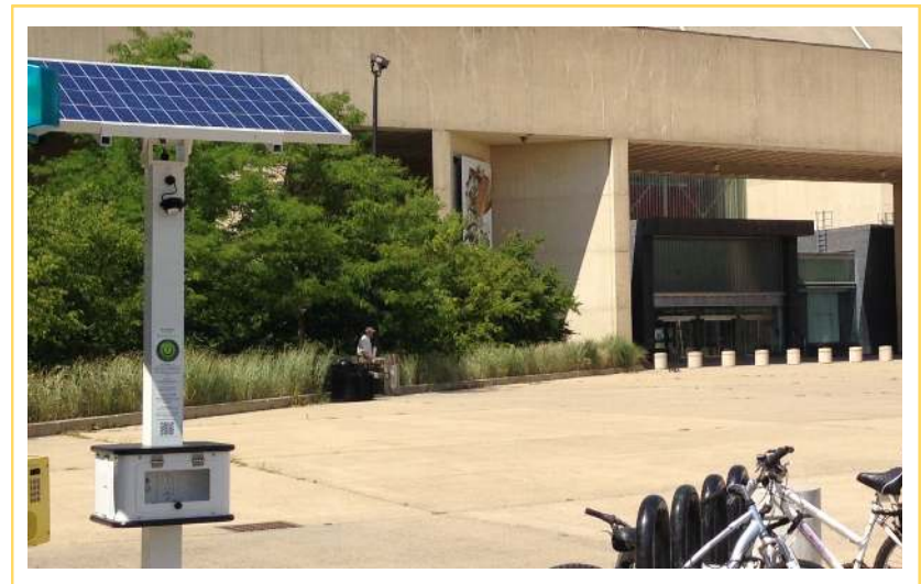
Solar powered device charging station. Source: University of Massachusetts Amherst
