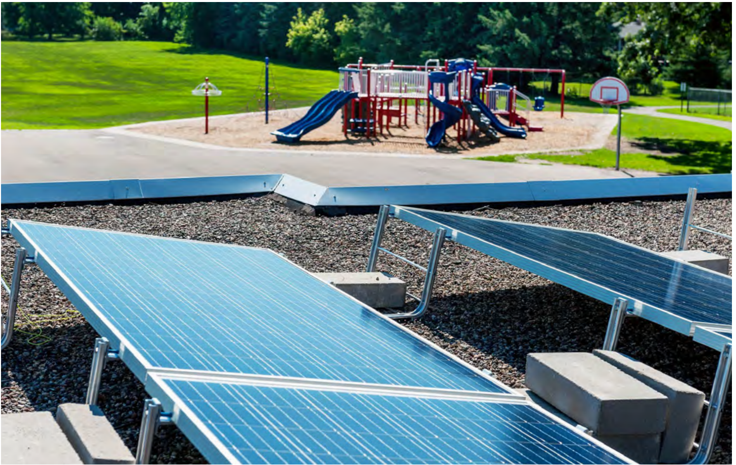
SNAIL LAKE KINDERGARTEN CENTER, SHOREVIEW, MN | CREDIT: IPS SOLAR
